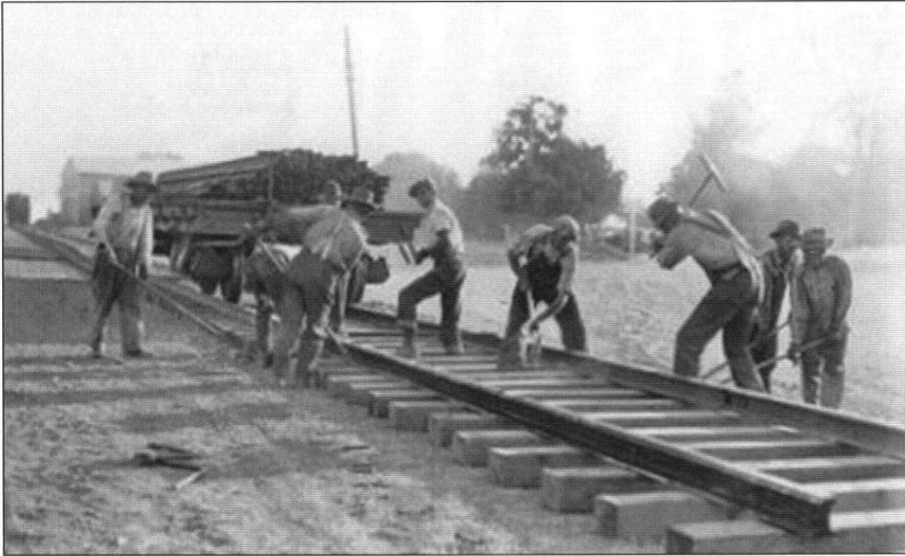
Crews built a five mile rail spur to the Pardee Dam construction site in 1928, confirming the importance of the Kentucky House line. Historical Society photograph.
