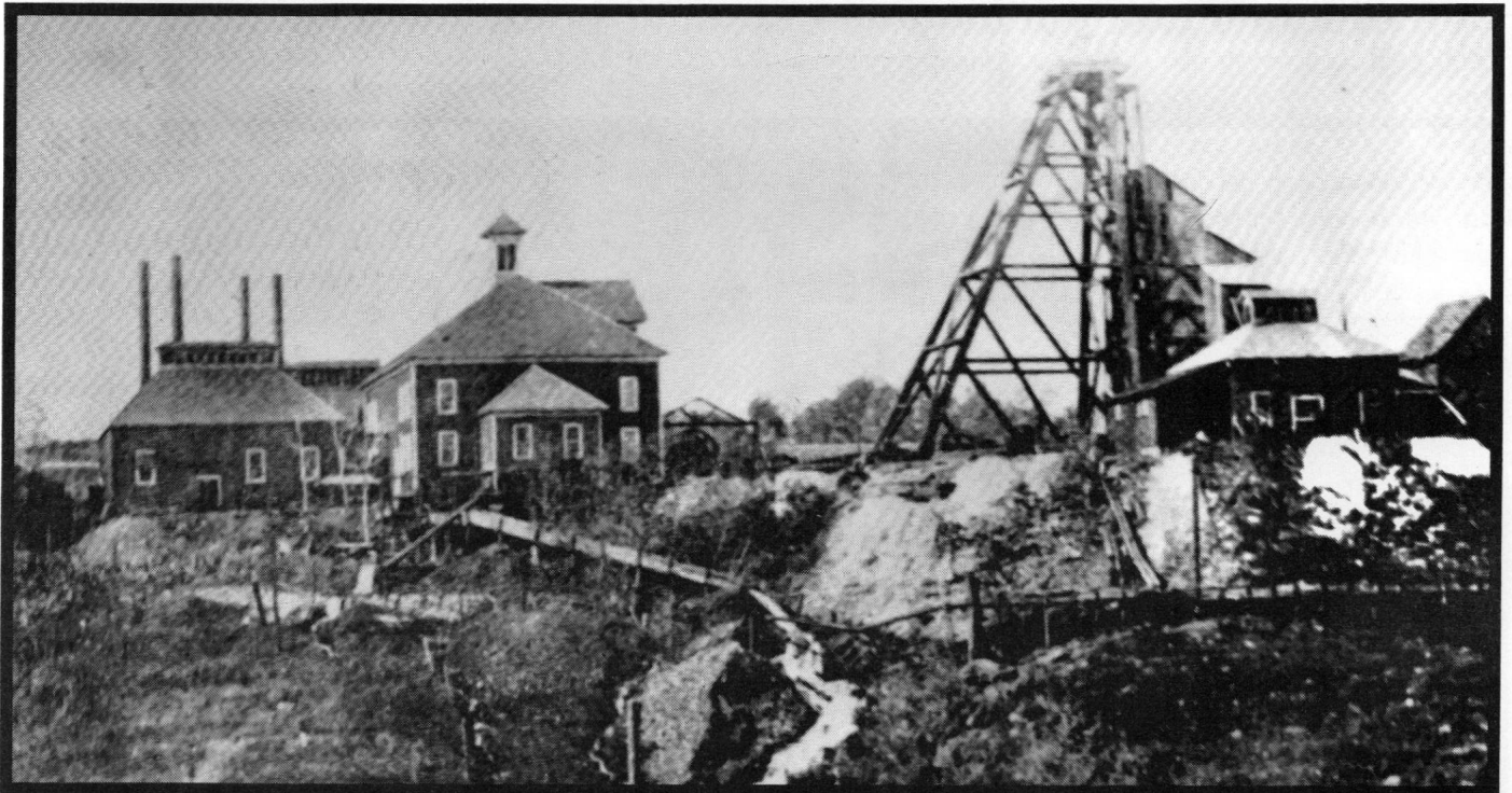
The Utica Mine Cross Shaft was on top of the hill behind the present Veterans' Building.
