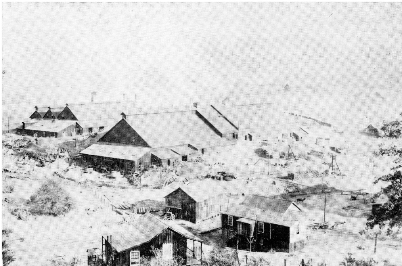
THE CHLORINATION WORKS
