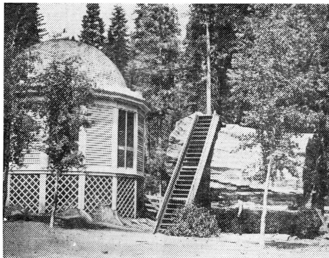
THE STUMPHOUSE —This house on the stump of the Big Tree cut in 1853 was used for many purposes. In 1858 for a period of four months the Big Trees Bulletin and Murphys Advertiser was published in it. The house was crushed by snow in the winter of 1917 and removed by workmen in the spring.
