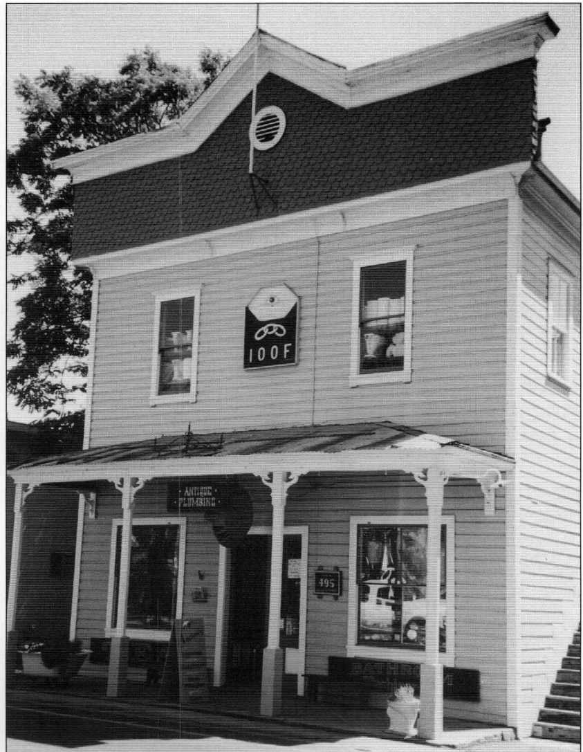
The IOOF hall built in Murphys in 1903 houses an antique plumbing supply business today. Photo by Bonnie Miller.
