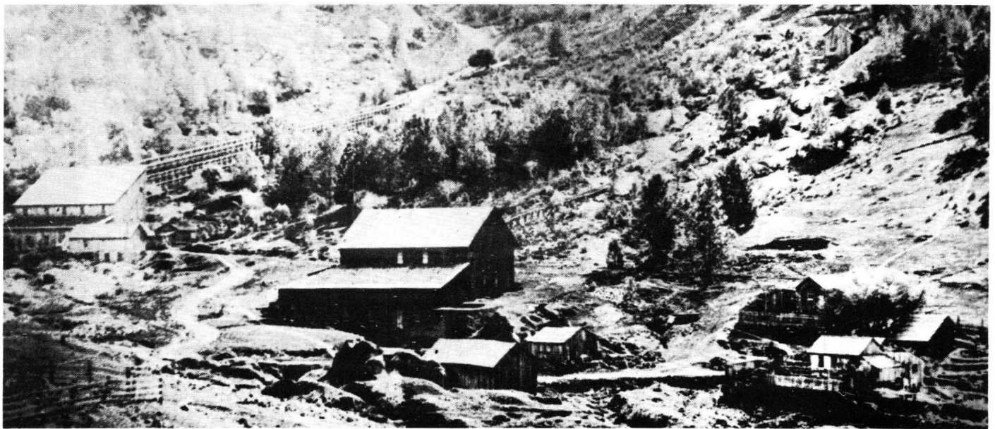
Reserve and Union Mines. Downhill tram brought ore to Reserve Mill, on left.
