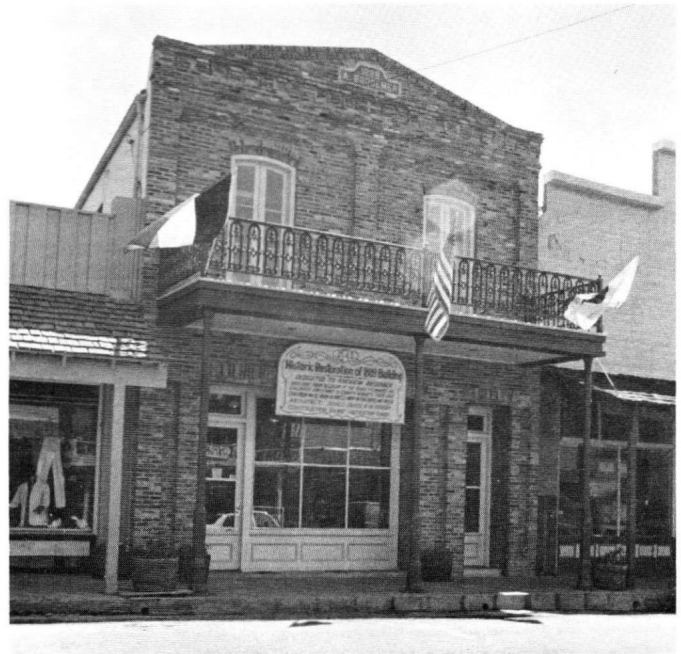
Brosemer Building, Main Street, Angels Camp
