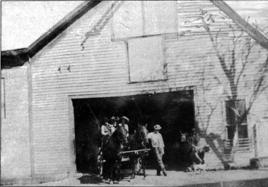
WASHBURN CARRIAGE HOUSE Across the street from the horse stable, this building, housing the carriages, was almost identical to the stable. Will O'Connell stands beside the Haupt team, with Louis and his daughters on board.
