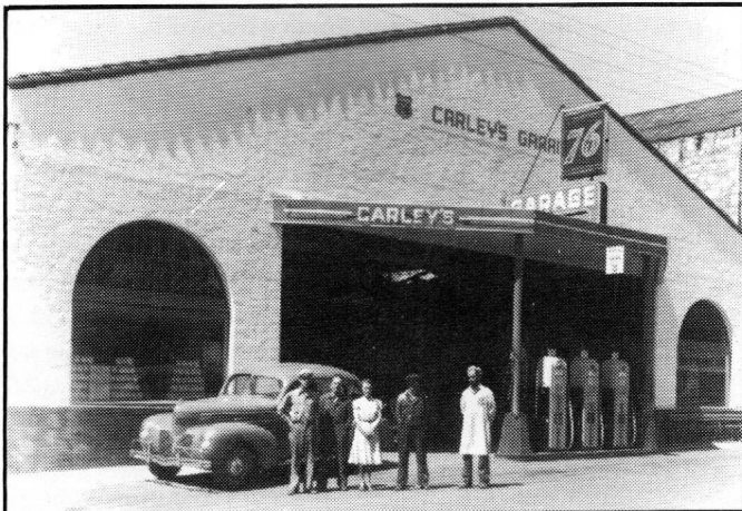
THE NEW GARAGE
