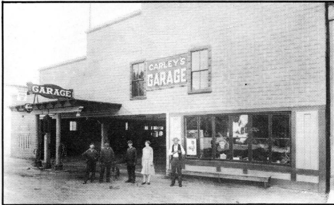
CARLEY'S GARAGE AFTER
