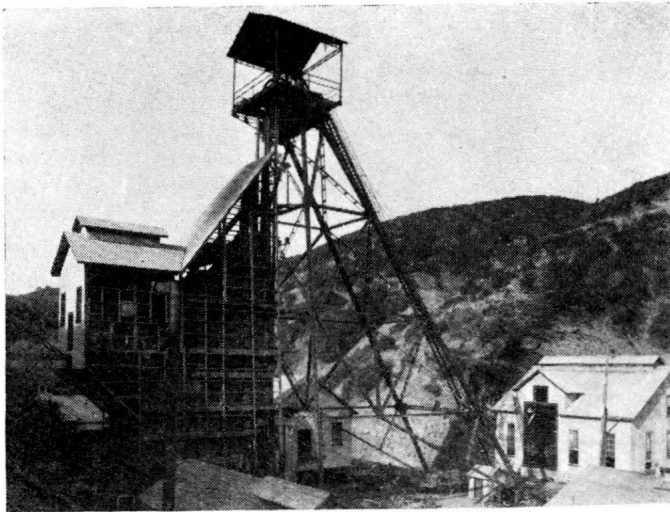
EARLY LANDMARK — Photo shows gallows frame of the Gwin Mine, just north of the old town of Rich Gulch, one of the early quartz locations in Calaveras County.
