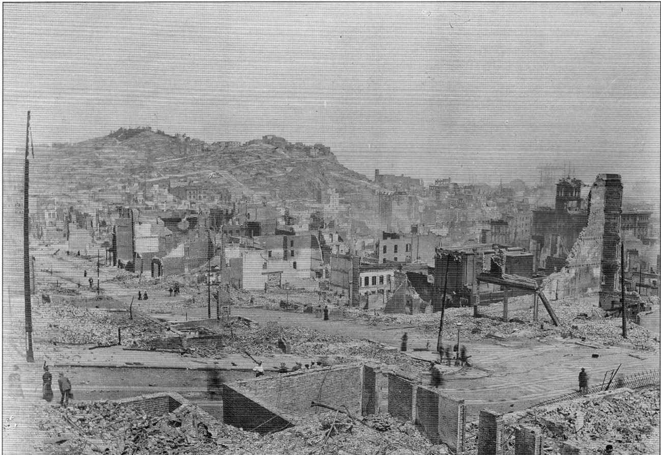
Little is left in the vicinity of Chinatown and Telegraph Hill; view is from above California and Stockton Streets. Masts of docked ships can be seen behind the steeple of the collapsed Hall of Justice.
