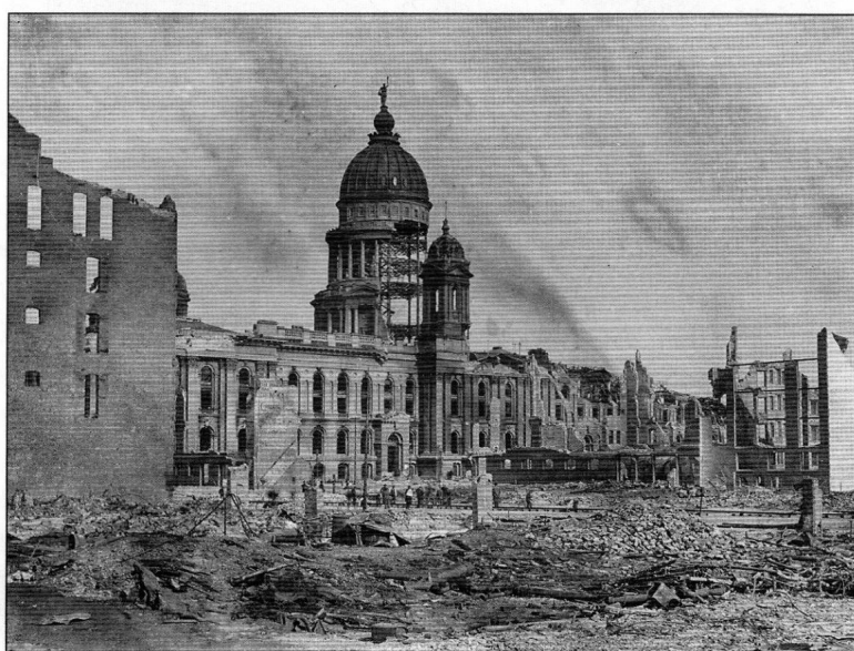
A view of the destroyed City Hall and its environs. It took 35 years to build at a cost of over $6,000,000 and toppled and burned in one day.
