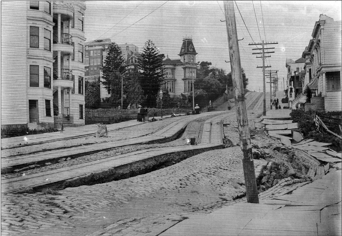
The fluid nature of the shifting fault lines shows up dramatically in this view up Union Street west of Steiner Street.
