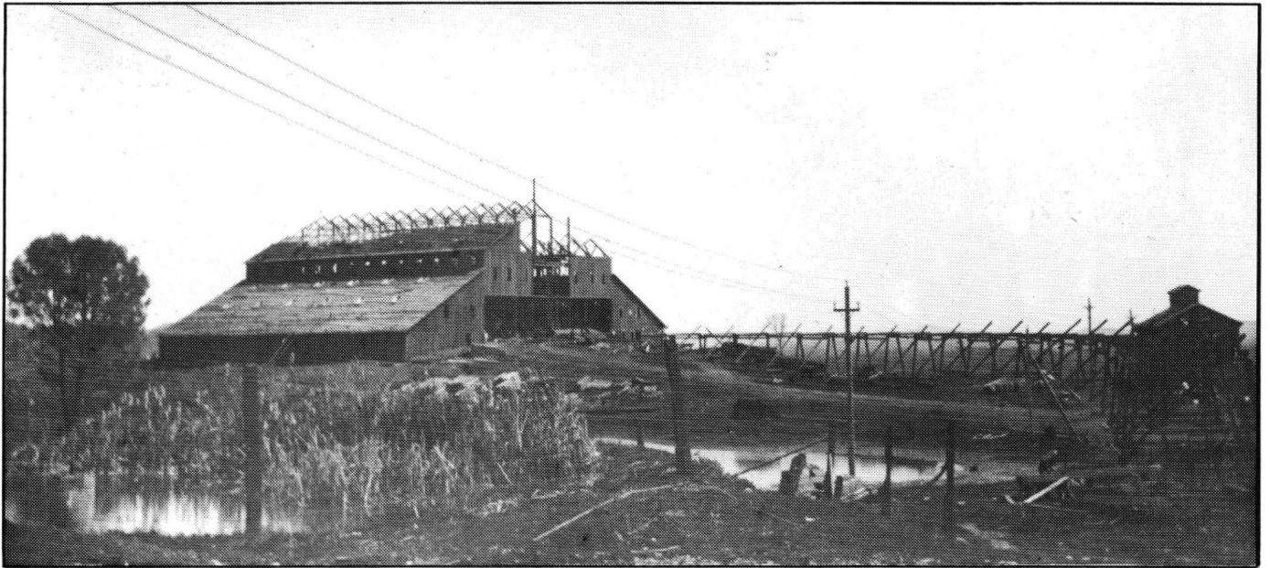
THE ROYAL MILL UNDER CONSTRUCTION
