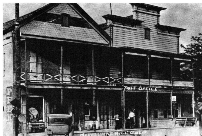
The Mokelumne Hill Post Office building as it appeared during the 1930s. The top floors were removed after 1946 explosion and fire.
