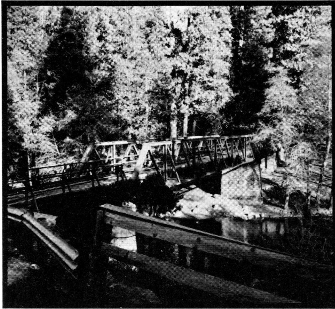
Bridge now replaces cattle ford at Board's Crossing.
