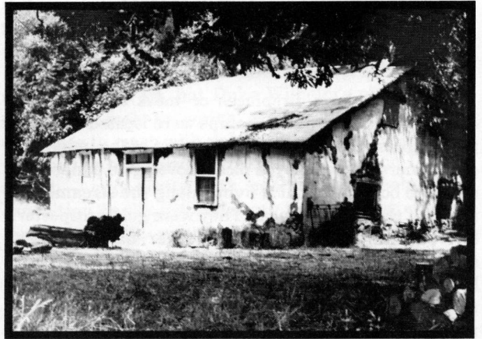
This stone and adobe structure was once the center of a thriving French enterprise on the North Fork of the Calaveras River.
