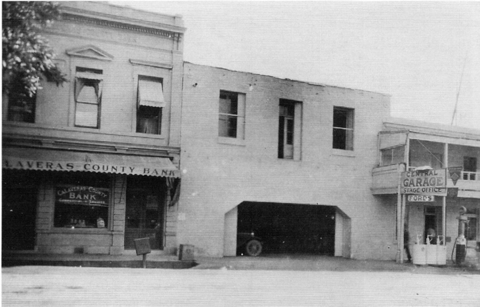
The Stickle Building in Angels Camp as it appeared around 1926. The original Stickle Building is the building on the right with the porch, built in 1856. The building in the middle, the garage with the archway, was built after 1900. Both buildings were built by Italian stone masons and still stand today. The building on the left was built by contractors from San Francisco and still houses a bank today. Note the gas pumps in front of the depot and the dirt street. Photo courtesy of Rene Baylor Photography.
