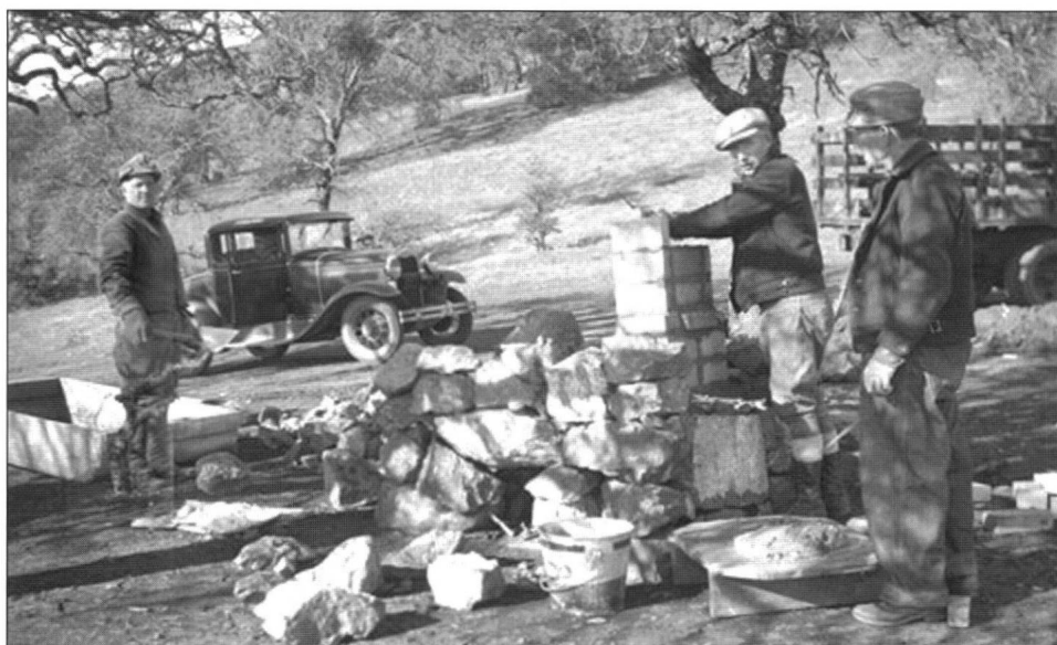
The CCC crew that worked at the Big Trees in the summer worked at Mt Diablo in the winter. Here the Mt Diablo crew builds a stone camp stove, circa 1939. Photo Courtesy California State Parks.
