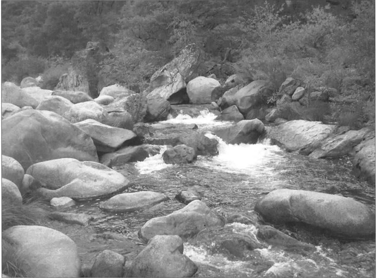
Footings of the former bridge built by the CCC are still visible on the Oxendine Trail.
