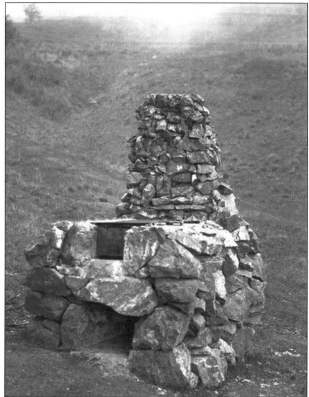
The Diablo camp stove, made of stone native to the sight, became a signature CCC improvement found in state campgrounds. Photo courtesy California State Parks.
