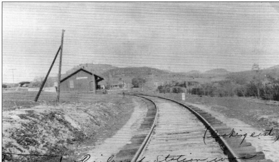
Helisma, Railroad Station at Burson, circa 1917. Calaveras County Historical Society.
