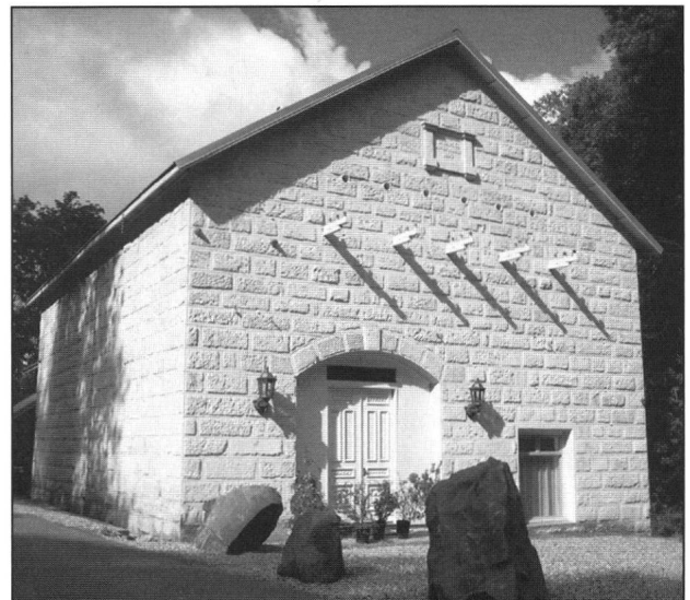
The mighty Utica Powerhouse is no longer an eyesore and once again graces the side of Utica Powerhouse Road in Murphys.
